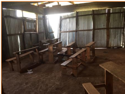
Iron sheet walls need replacement
