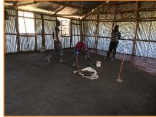
Staffroom being prepared: levelling before adding the sand cement mix
