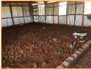
Staffroom being prepared: levelling before adding the sand cement mix
